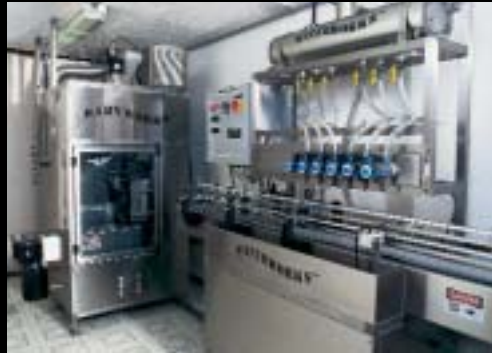
Custom Electrical, Plumbing, Insulation Installation
